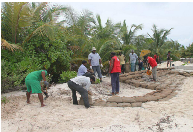
Kolhufushi volunteers active in building cement bag barrier around the island
